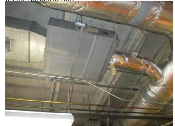
*Figure III-6. Existing pneumatic VAV terminal unit.*
