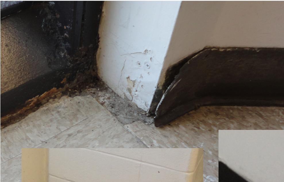
Wall Base – Sections of resilient base are loose or missing in several areas. Many rooms with CMU partitions and concrete floors have unnecessary resilient base.
