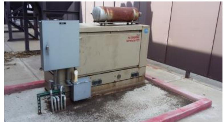
Figure VI-2. 40 KW Diesel Generator.
