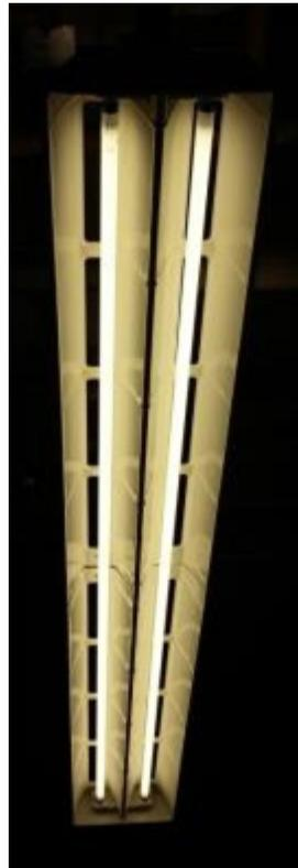
Figure VI-7. Typical 8' Strip Luminaire
