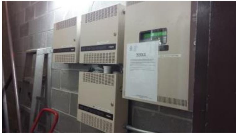
Figure VI-12. Existing Fire Alarm Control Panelboard.
