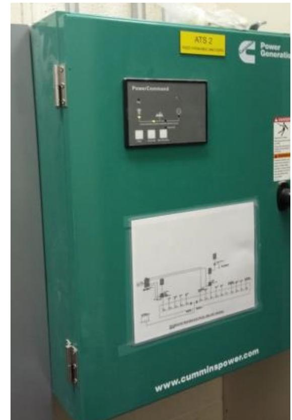
Figure VI-5. Automatic Transfer Switch #2
