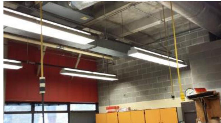
Figure VI-10. Typical Lab Cord Drop Receptacles.
